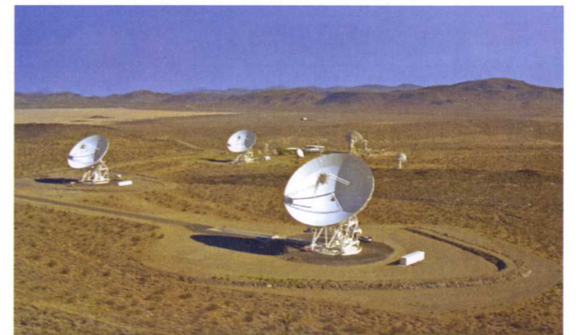
BELOW Three 34m (110ft) diameter Beam Waveguide antennas located at the Goldstone Deep Space Communications Complex, situated in the Mojave Desert in California. This is one of three complexes which comprise NASA's Deep Space Network (DSN). (NASA)
