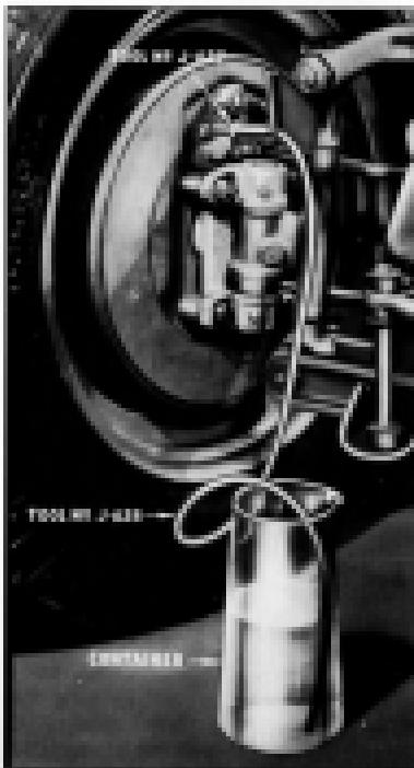
Fig. 171. Brake Bleeding Operation.
